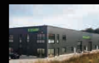
Germany Aachen R&D Center and Technical Center
